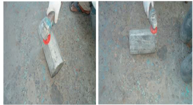
FIGURE 6: Grinding of columns.
